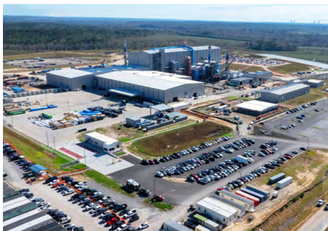
The Aurubis Richmond site at the start of December 2024.
