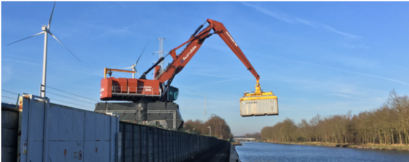
Ship loading facility (Cu-Port) at the Olen site
