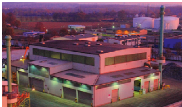
Aerial photo of the material preparation, crushing, and separation plant (MV-ZS facility) in Lünen
