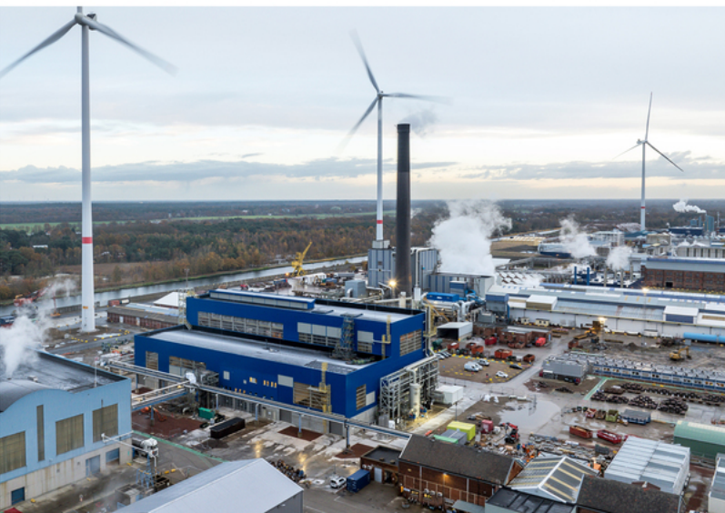
The BOB facility at the Olen site.
